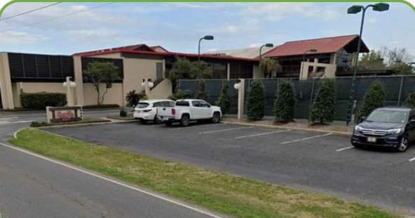
Possible Parking lot encroaching in R/W
