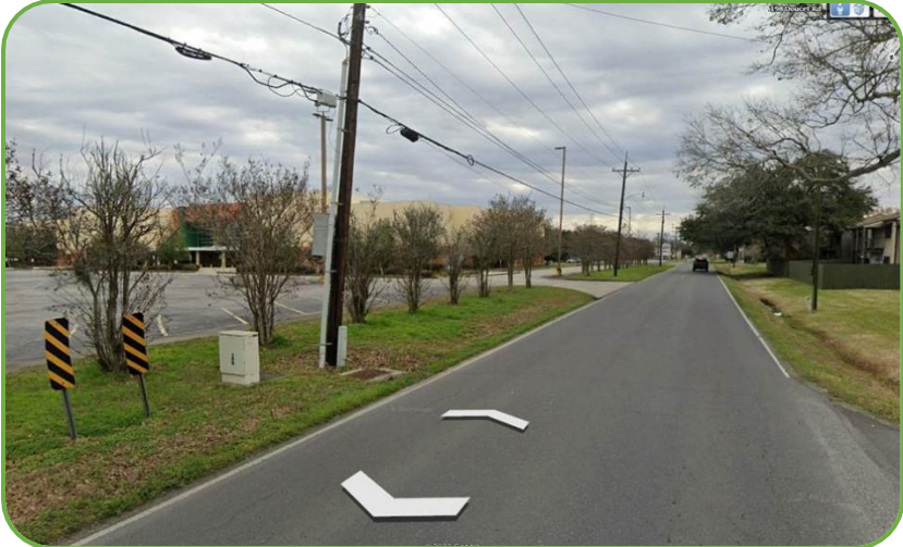
Utilities and Drain Inlet Near Road
